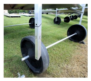
4. Draw a line where you want to cut off the leg, copying the same angle as the original leg bottom. Use a reciprocating saw to cut off the portion of the leg you wish to remove. Bonus points if you clean up that edge with a file! Then drill a 3/8" hole, the same distance from the new bottom of the leg as the hole in the original leg bottom.
