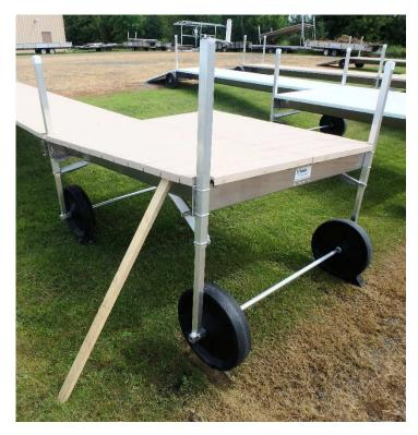
2. Wedge a 2" x 4" at an angle between the ground and the <u>aluminum lip</u> on the V-Beam near the leg that needs to be shortened. (Not the plastic decking.)
