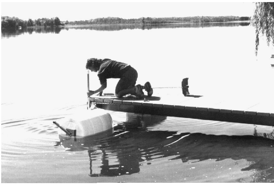
6. (Remove handle) Roll dock section into place & secure post in post bracket.
