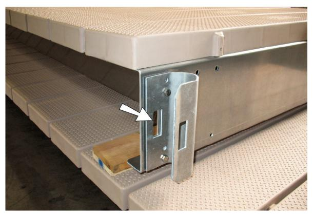
Place the post bracket on the end channel as shown. Make sure the square hole on the post bracket & the end channel are alligned. Fasten with (2) 5/16" x 3/4" hex head bolts & flange nuts
