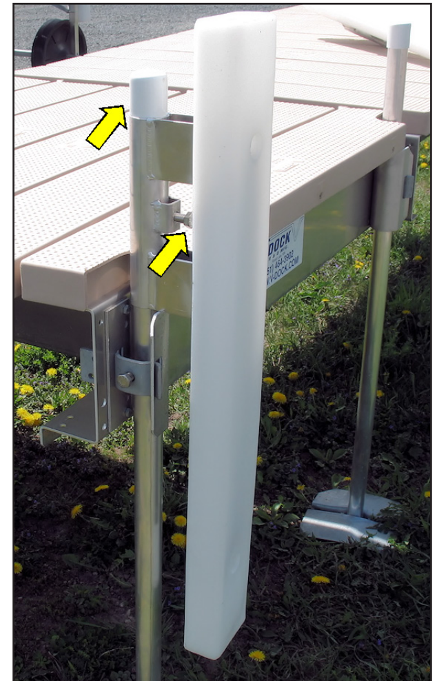
Tighten set bolt and put post cap back on.
