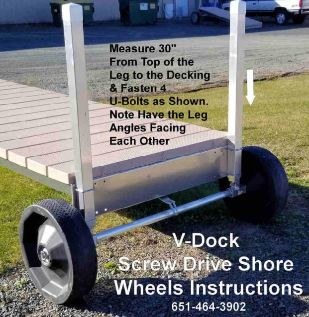
Slide the axle connection into the leg as shown. Tighten the spring bolt and lock nut until the theads of the bolt just goes beyond the lock nut leaving the spring flexable.
