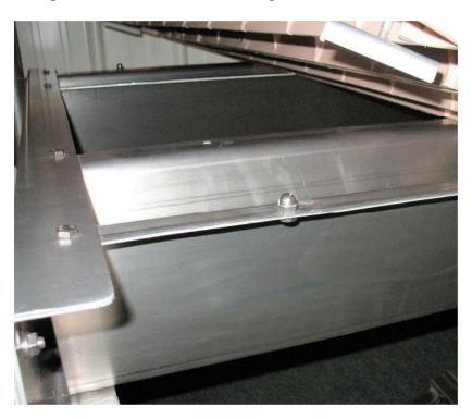
Next, install reinforcement tabs on the left and right side of the shore end channel, where you removed the decking in the previous step. Remove both 5/16" bolts and nuts, install tabs, and re-secure nuts and bolts as shown.
