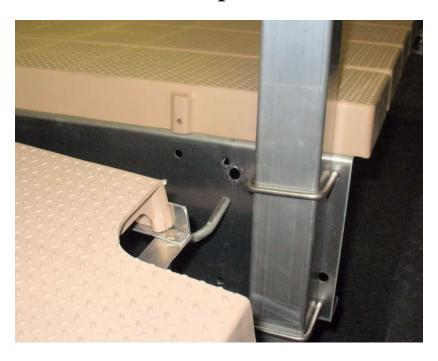
Slide the ramp off and remove the first deck panel on the shore end of the dock.
