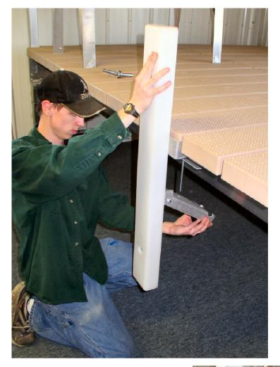
Next rotate bumper upright and swing the bottom arm so it grasps the bottom of the V-beam. Fasten carriage bolt & flange nut.
