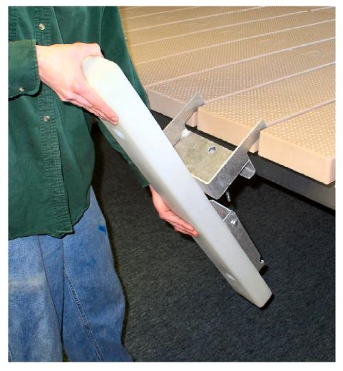
Insert vertical moveable bumper in between the board slats and onto V-beam. This can be only fitted where there is not a crossmember on the V-beam.
