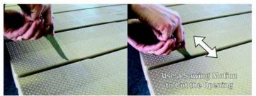
Saw towards to outside edge. At the end of the tab you will hit the V-Beam and need to saw a little on top of the V-Beam to finish cutting the tab.
