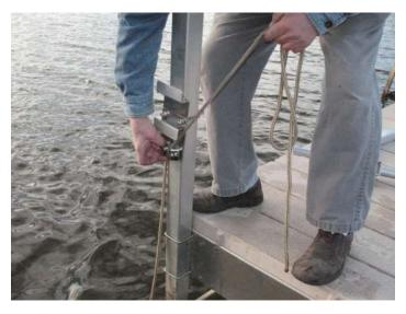
10. Pull the rope through the quick-locking cleat.
