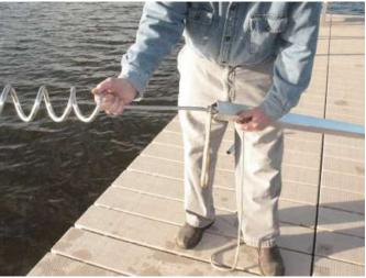
3. Pull the rope snug and feed the spiral anchor loop into the bottom of the installation T-Bar. The loop fits into the bottom of the T-Bar diagonally. Tap it gently on the ground to lock it in snugly.
