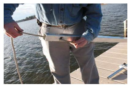
2. Thread the rope from anchor through the hole at the bottom of the installation T-Bar.
