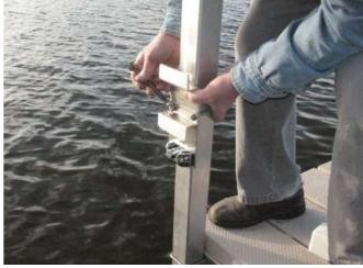
1. Crank the leg down approximately 6" lower where you would like to install the anchor. Slip the cleat bracket onto the leg and tighten it into place about 12" to 18" above the decking.
