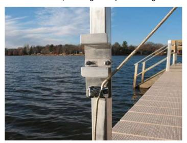
11. Step back and pull the rope taut. Adjust the height of your dock back up to the desired level.
