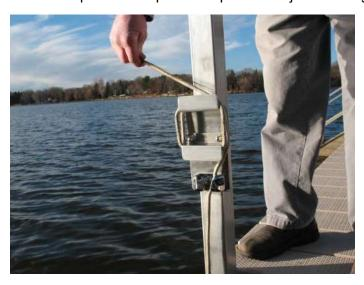
12. Wrap the excess rope around the tabs of the cleat bracket.
